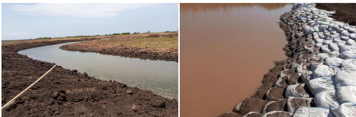
***FIGURE 4: A BIOSWALE CONSTRUCTED BY DRC TO HARVEST EXCESS WATER-LEFT AND SAND PACKED IN NYLON BAGS TO PREVENT WATER FROM CUTTING THE SOIL.***
